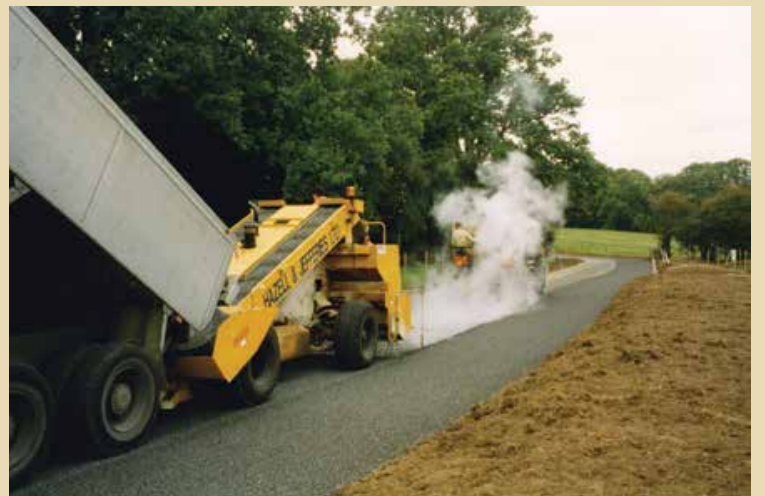
White limestone formed the foundation of the 1 kilometer long driveway. Together with highway landscaping at the new entrance, the roadworks were completed in record time.
