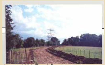
August 1996 (Road Construction)
