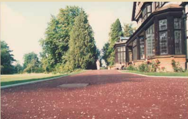
The Manor was given this fresh perimeter path of red tarmac
