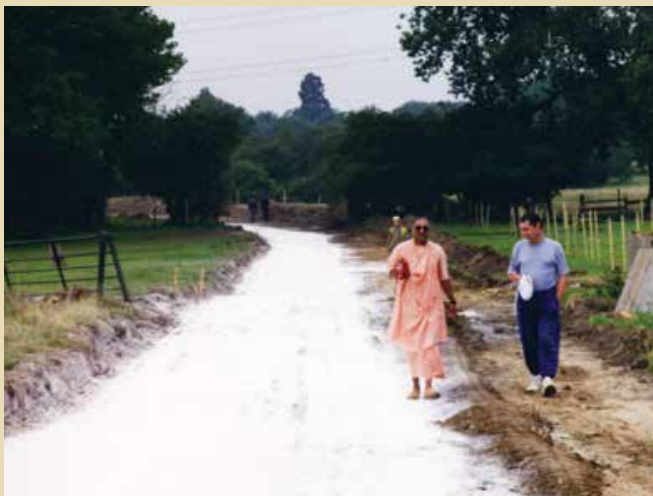
White limestone formed the foundation of the 1 kilometer long driveway. Together with highway landscaping at the new entrance, the roadworks were completed in record time.
